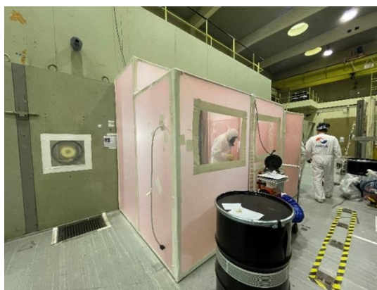
Ispra - Ontsmetting van hete cellen in LCSR
