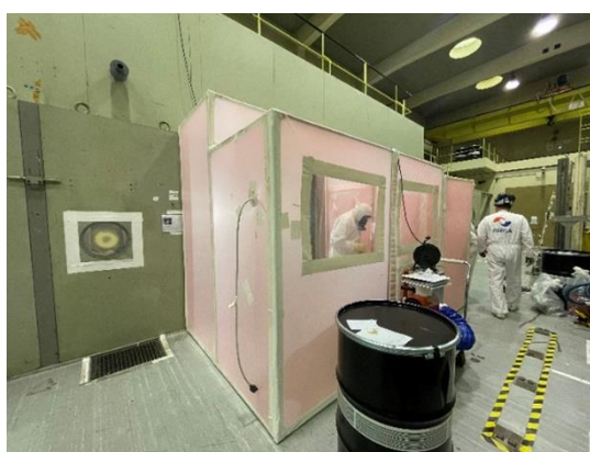
Ispra-Decontamination of hot cells in LCSR
